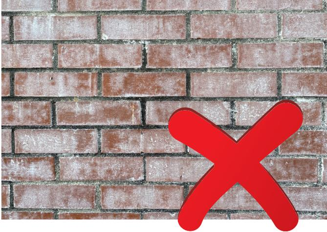
*Try 50% mix of white vinegar and water to remove persistent efflorescence with a rigid brush following cleaning with a pressure washer, allow to dry and apply in dry conditions for upto 72 hrs before washing off. \**
